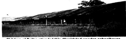
Children of Belize attended this dilapidated wooden schoolhouse.
