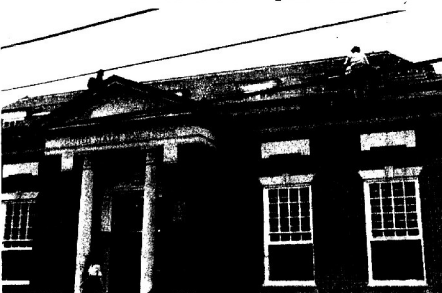
Those leaks which showed up recently in the post office roof here will hopefully be no more with a new roof job being completed. The structure has undergone extensive repairs in recent weeks.
