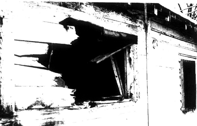
Portion of Riverside apartment building which suffered the direct hit in Saturday night's dynamiting.
