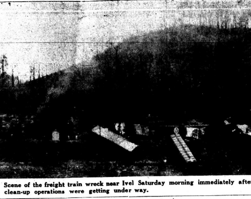
Scene of the freight train wreck near Ivel Saturday morning immediately after clean-up operations were getting under way.
