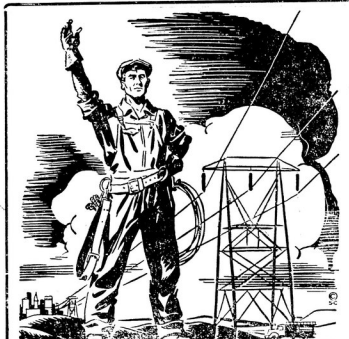
Electrical Construction Contractors Erectors of power and telephone lines.
