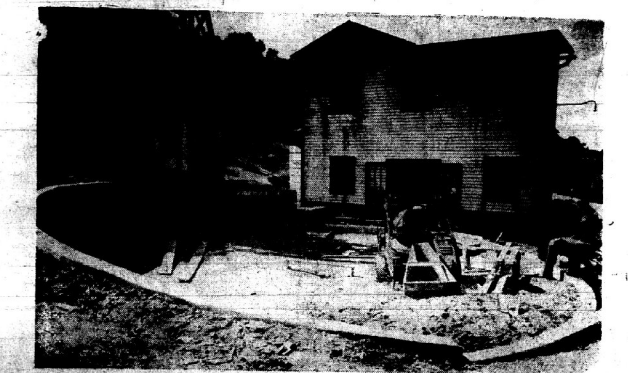
That isn't a trench mortar looking at you—it's a concrete mixer in operation at Wheelwright on the construction of a new filter plant, one item in a $150,000 sanitation project. (Additional pictures on page five).
