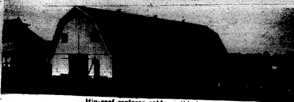
Hip-roof replaces gable on this barn.
