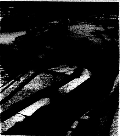
OLD MAN RIVER in miniature, rampages and all, is constructed by the U. S. Army Engineers at Vicksburg, Va., to learn vital flood control lessons. The laboratory covers 225 acres and includes an 80-acre lake. (Acme)
