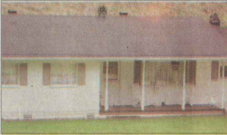
Nora Blair had replacement gutters, but no one to install them and no way to pay for installation. She found help at Big Sandy Area Community Action Program.
