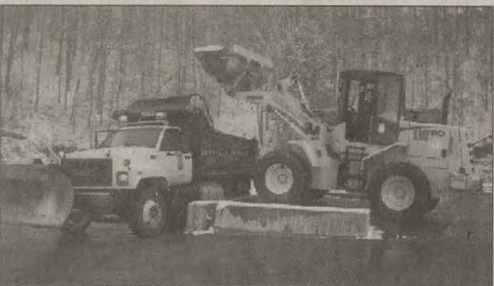
Re-loading a salt truck is just one of the many steps in snow and ice removal. Highway District 12 has more than 200 people involved in the process of battling winter weather, flooding, and other weather emergencies. (2) Inside lanes are cleared first, then outside lanes. Motorists should be respectful of the snow plow. They have to drive at a certain speed in order to spread the salt or liquid calcium chloride in the proper amounts. Don't try to pass it; the driver will pull over when it's safe to do so.
