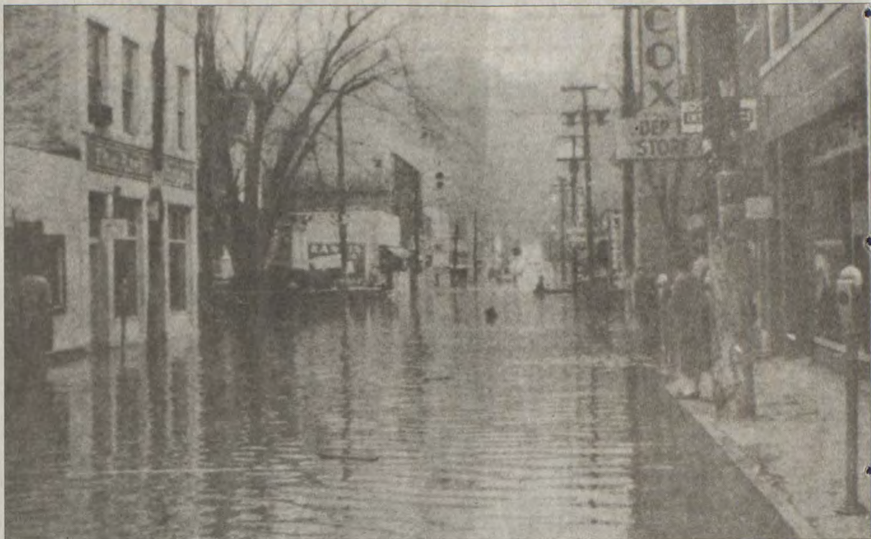
Flooding in downtown Prestonsburg, during the 1957 flood, one of the most destructive in the county's history.
