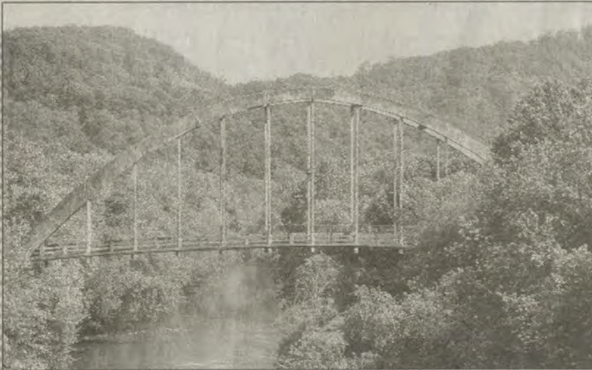
The West Prestonsburg arch bridge drapes across the Big Sandy River as a testament to engineering brilliance and creativity. Although no longer used as a primary means of travel, the bridge is a reminder of Prestonsburg past cutting edge construction efforts.
