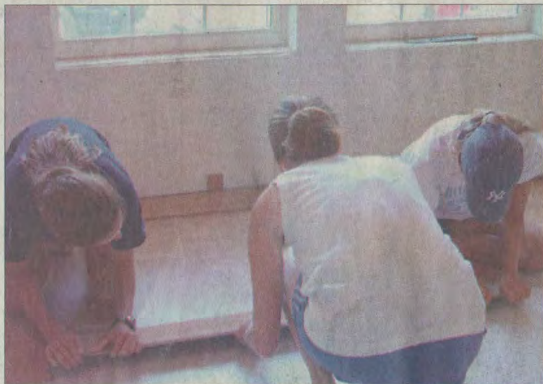
photos by Jessica Hale Above: Lexington First Presbyterian Church group members install laminate flooring, just one of the many finishing touches on the latest LINKS house. Right: The latest LINKS house is nearing the finish line as the Lexington Presbyterian Church pitches in to help this week. Floyd County Judge Executive Barry Davis is pictured with church group members Elizabeth McCorvey, Havana Childers, Hannah Goodman, Becky Goodman, Andrea Merchak, Perry Garrett, Randy Master and Claire Simon.
