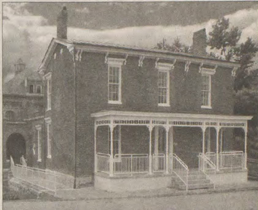
The newly renovated "Jailer's House," located at 117 N. Water St., in Georgetown, was built between 1875 and 1891. It now serves as the Scott County Arts and Cultural Center, housing a gift shop, offices, and arts studios.
