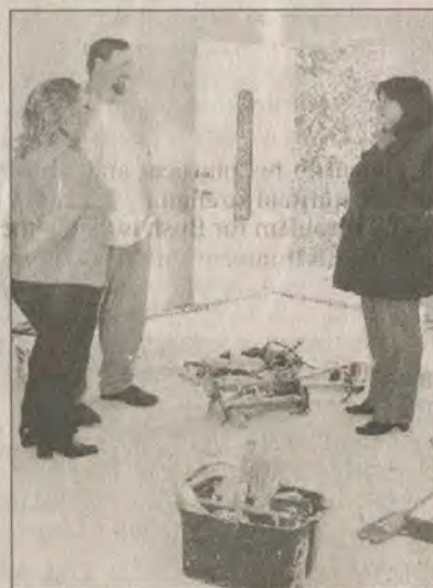
Joyce Wilcox, right, talks with Mark and Vicki McKenzie in the living room of the couple's new home going up near Inez. As Business Services representative for the Big Sandy Area Community Action Program, Joyce works as a liaison between Booth Energy and Excel Mining—the two sponsoring coal companies training and employing participants in the Coal Careers Program—and the Eastern Kentucky Concentrated Employment Program, Inc. (EKCEP), which helps fund the Coal Careers Program.
