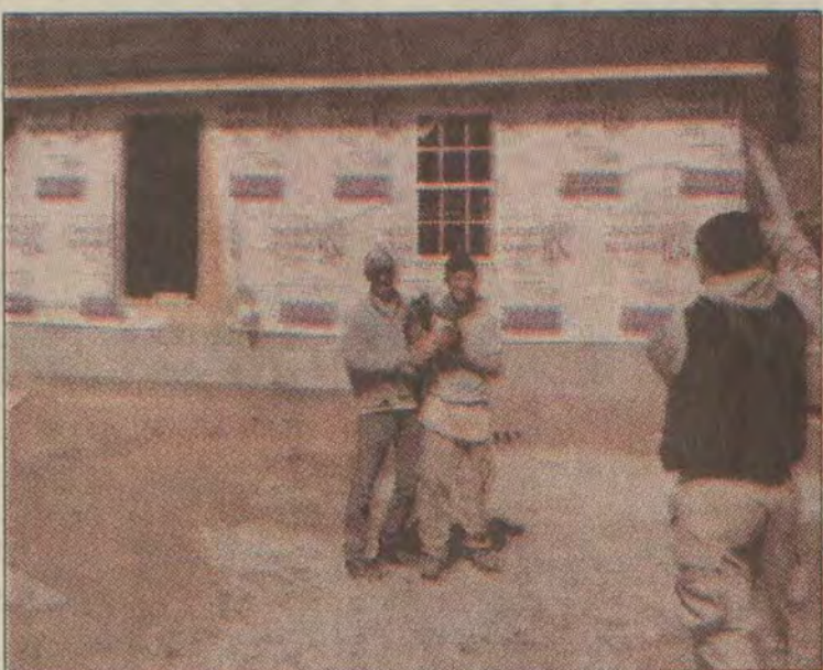
AmeriCorps*NCCC members pose with a local resident in front of the house they are building for a low-income client at Branham's Creek.
