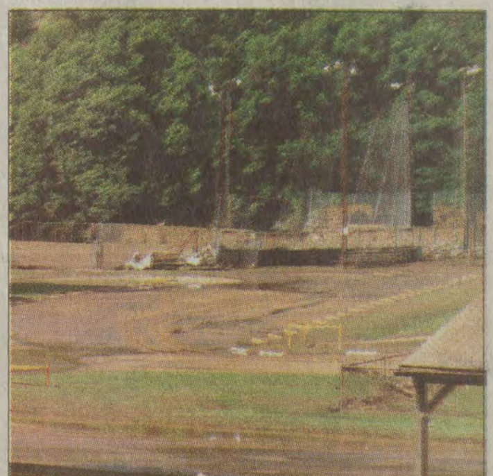
Dugouts were wiped out, left lying in the wake of flood waters.
