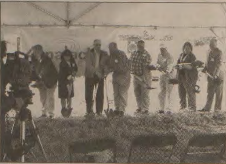
Company and local officials held a groundbreaking ceremony at the site of the new Appalachian Wireless headquarters at Ivel. When complete, the company will employ roughly 100 people at the site.
