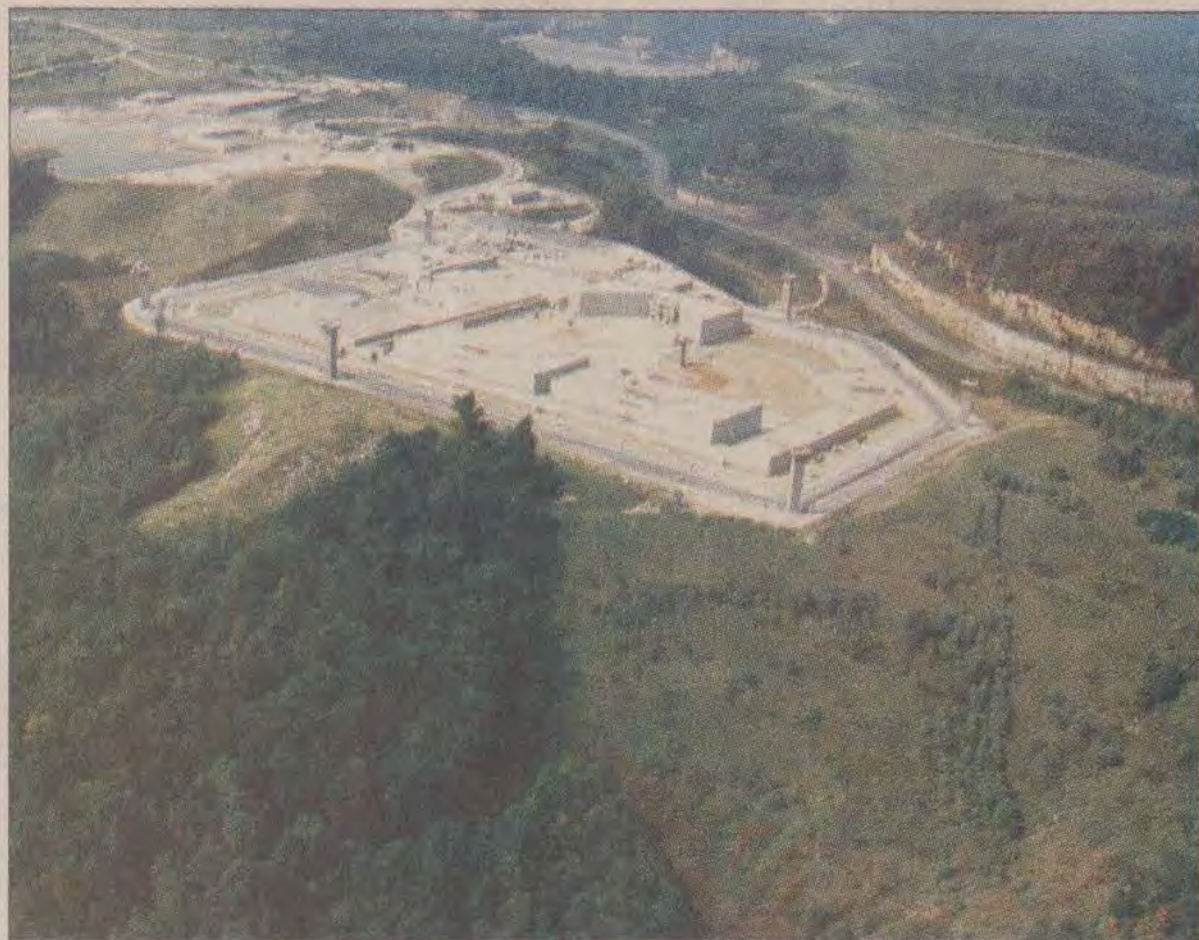
The Big Sandy federal penitentiary, shown above during construction last year, has missed two deadlines for opening and must continue to wait for Congress to adopt a budget before progress can continue.
