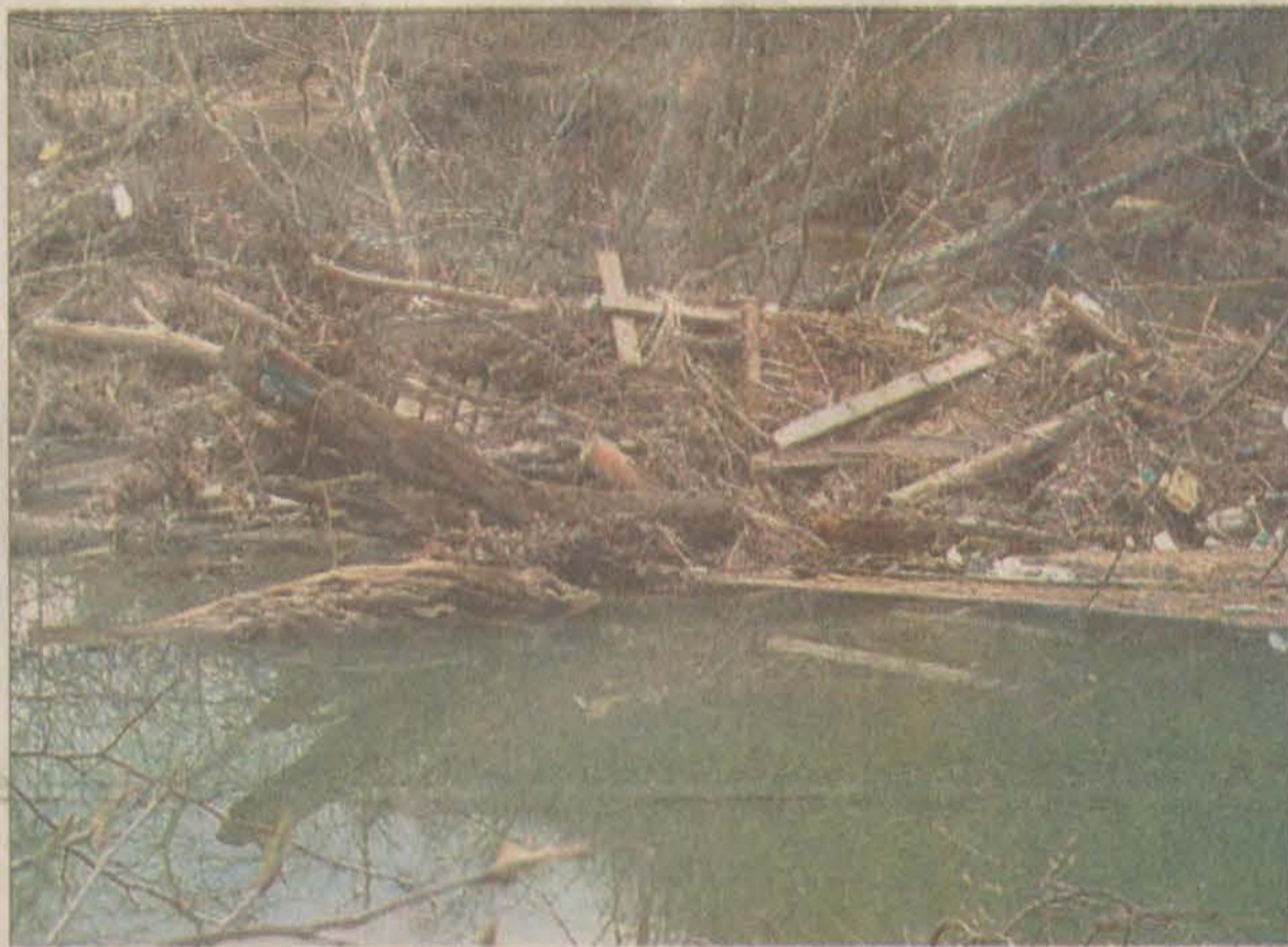
An unsightly combination of garbage and fallen trees has some residents along Middle Creek worried about the potential for flooding in that area.
