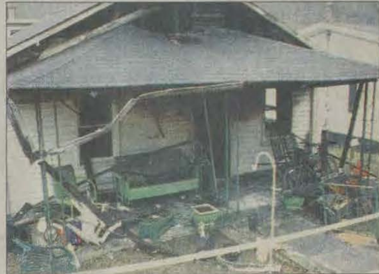
The remains of a house belonging to James Howell that burned this past weekend on South Highlands Avenue. Howell was killed in the fire.
