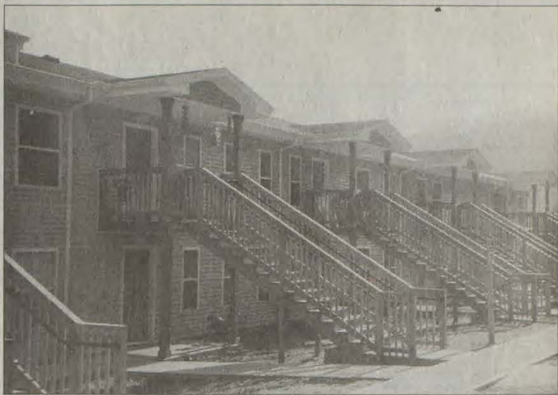
Jarnigan Place was constructed exclusively to house low-income families.
