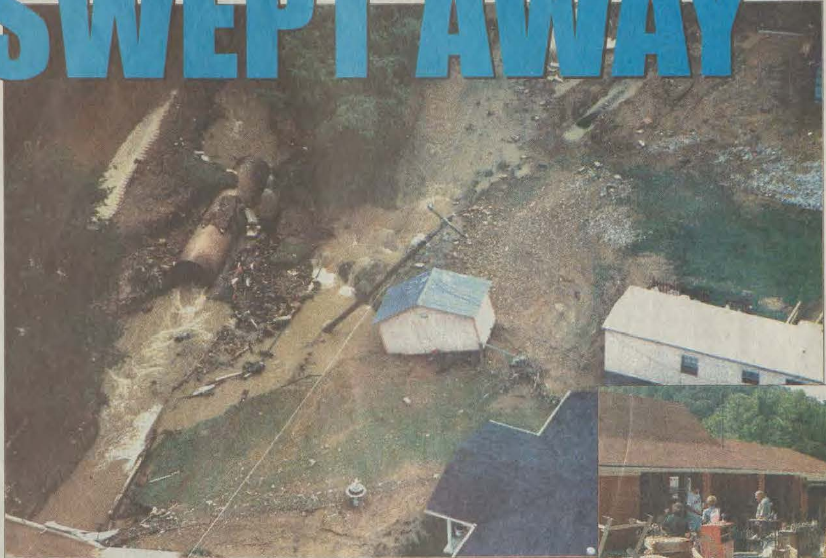
An aerial view of Tinker Fork, left, shows the wide-spread damage raging floodwaters caused to anything in their path. Bridges, buildings and roads all gave way under the tides, causing millions of dollars in damages and resulting in disaster declarations by County Judge-Executive Paul Hunt Thompson and Gov. Paul Patton.
