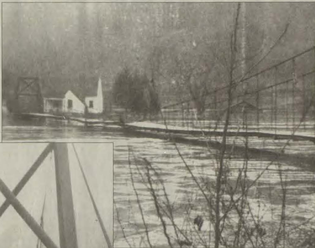
The bridge, with a damaged middle after being struck by a house washed away upstream by flood waters.
