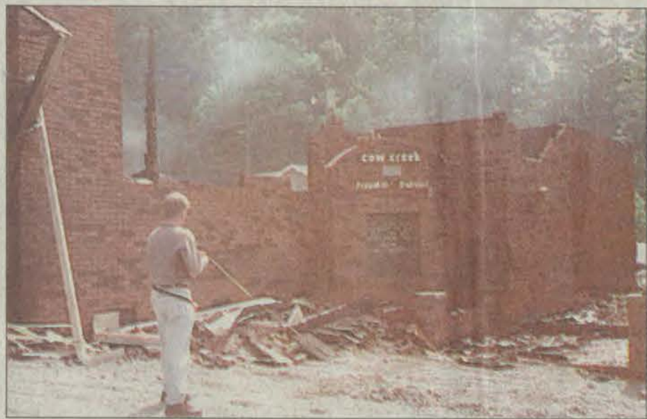
photo by Ralph B. Davis An insurance adjuster surveyed the damage at Cow Creek Freewill Baptist Church Tuesday morning. The building, constructed in 1933, was expected to be a total loss.
