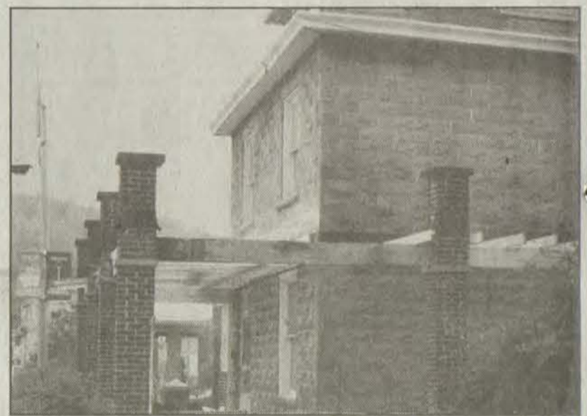
Renovation of what is now the Ramey Insurance building began last year with replacement of the porch. The building is believed to have been constructed in the early 1900s.
