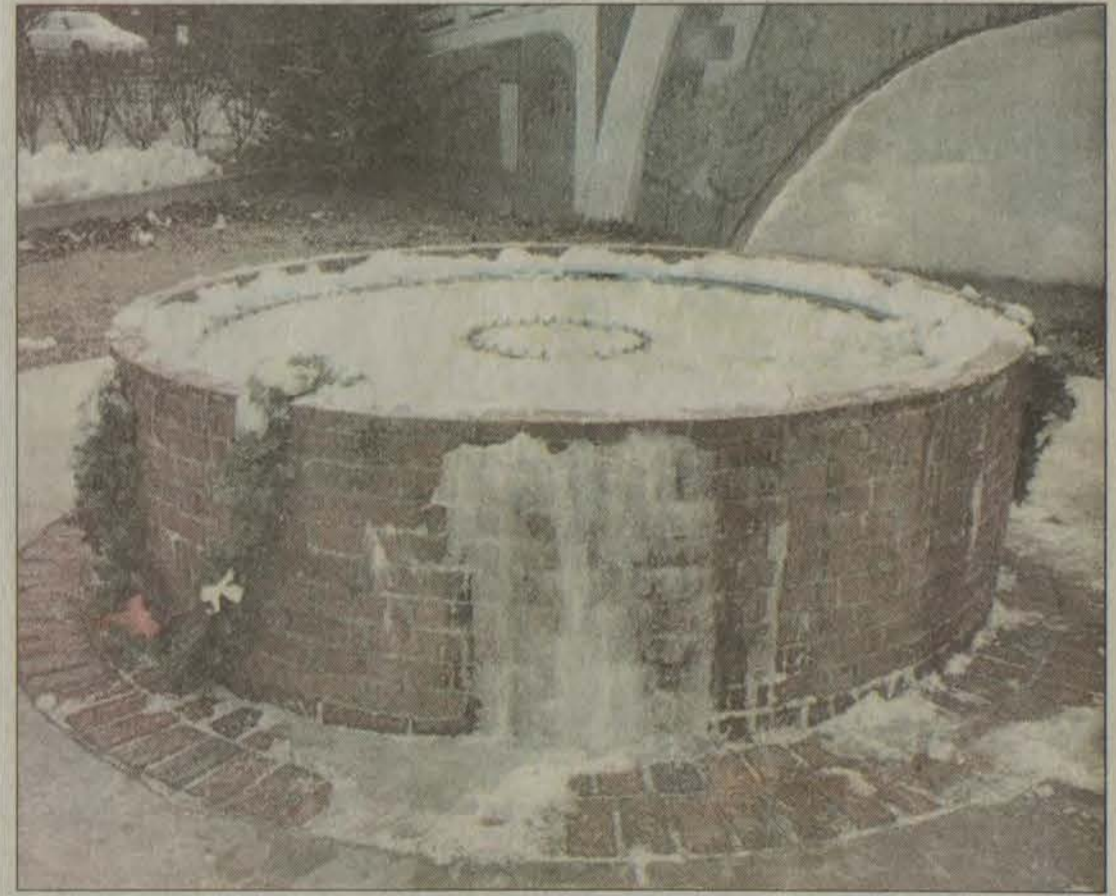
"Old Man Winter" blew some gusty breaths over and across the city's downtown fountain in the past few weeks, leaving, at one point, cascades of water frozen in midstream. Public Works personnel went to work on Thursday afternoon, chipping away large chunks of the ice, seen laying in the background. Jack Frost is also not done with Floyd County, with forecasters predicting snow over each of the next four days.
