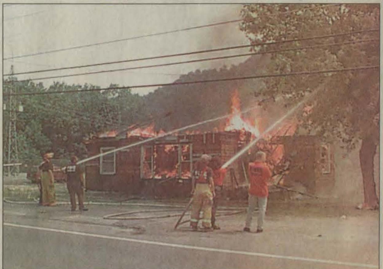
Kate Gullick and Rebecca Rowe were among the firefighters participating in a fire training session Friday on South Lake Drive near Calhoun's Garage. Their duties included hosing down a tree in front of the building and the nearby Calhoun's Garage. (photo by Janice Shepherd)
