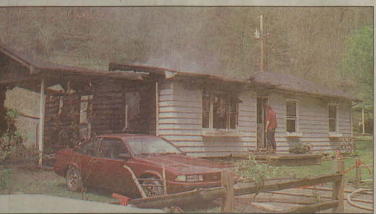
The home of Ron and Ruth Shortridge of the Jack Arnett Branch community was destroyed by fire Wednesday. The Middle Creek Volunteer Fire Department responded to the blaze. The Shortridges' son James lost his first deer that was mounted in the living room in the blaze. The Shortridges said they had only enough insurance to pay off the FHA loan on their home. Firefighter Jeff Shepherd said the items left in the unburned portion of the house would not be usable. The cause of the blaze is not known and remains under investigation. (photo by Willie Elliott)
