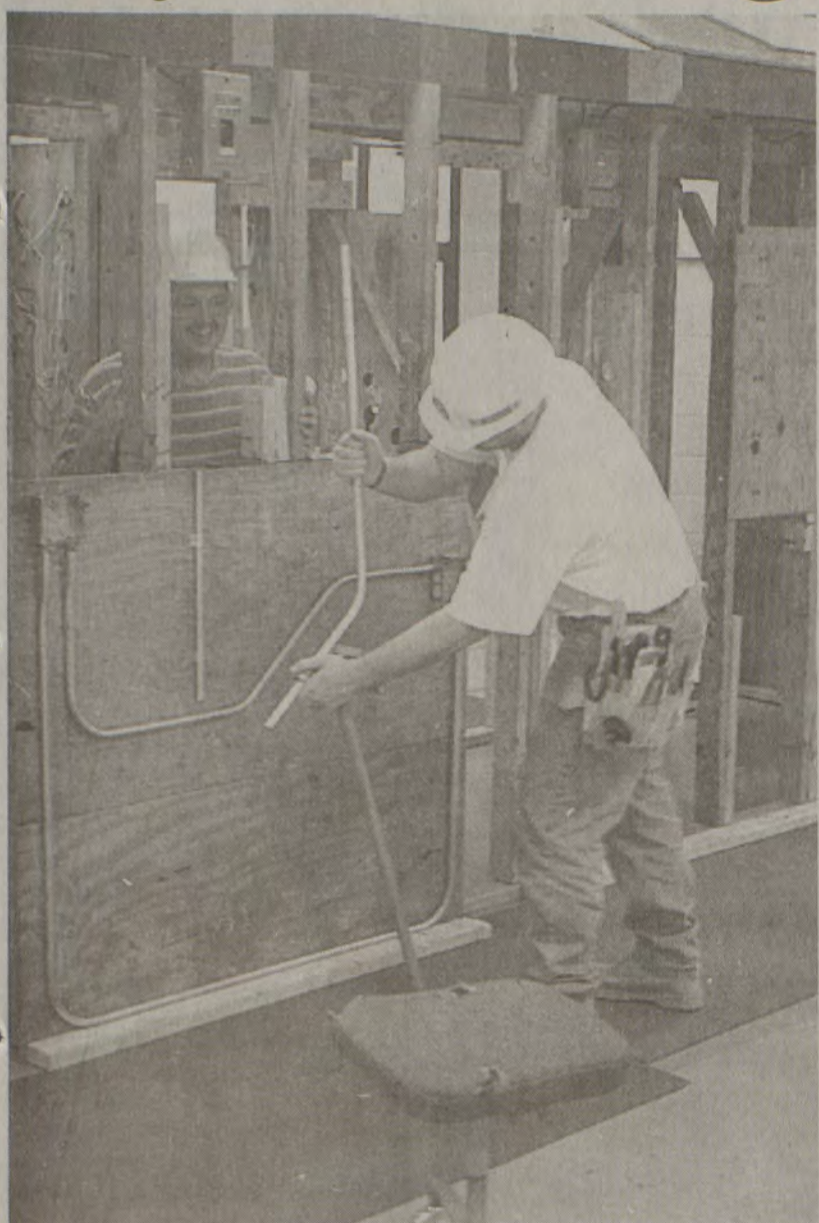
As one student worked with conduit at the college's Paintsville campus Friday, another observed the delicate procedure. The Electrical Industrial Technology class teaches students construction wiring in accordance with the National Electrical Code.
