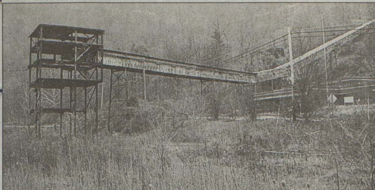
The tippel at Price stands as a reminder of the days when coal was king. The tippel served major coal companies such as Inland Steel and Island Creek plus local coal producers. Much of this plant has been dismantled, but this section stands as a symbol of the better days of coal mining in eastern Kentucky. (photo by Willie Elliott)
