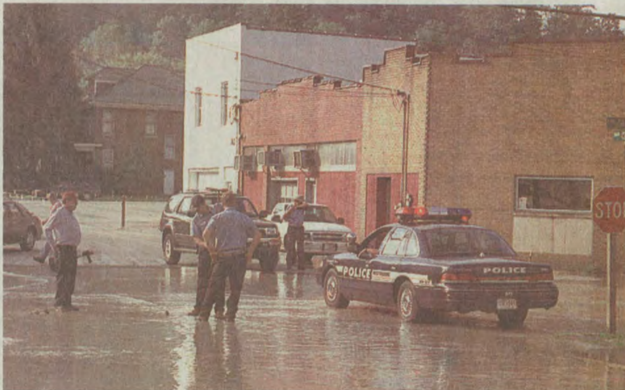
City utility workers waded through water Thursday morning while trying to turn off a water line which flooded Graham Street. Seldon Horne, with Prestonsburg Utilities, said a section of the water pipe began leaking because of "severe corrosion." Approximately 100,000 gallons of water was lost because of the leak, Horne said. (photo by Chris McDavid)
