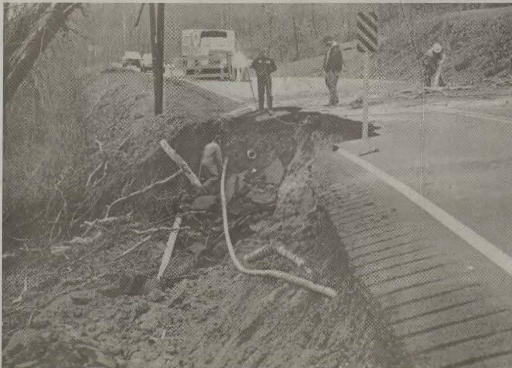
Route 122 on Left Beaver (above) was covered in several places and eventually closed to traffic. In Johnson County, a slide cut out a portion of Route 40, exposing a live gas line (left).
