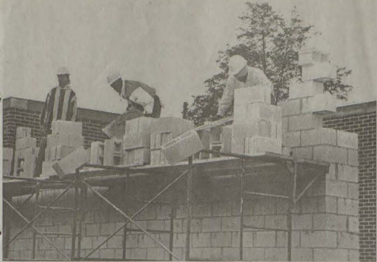
Building a wall
