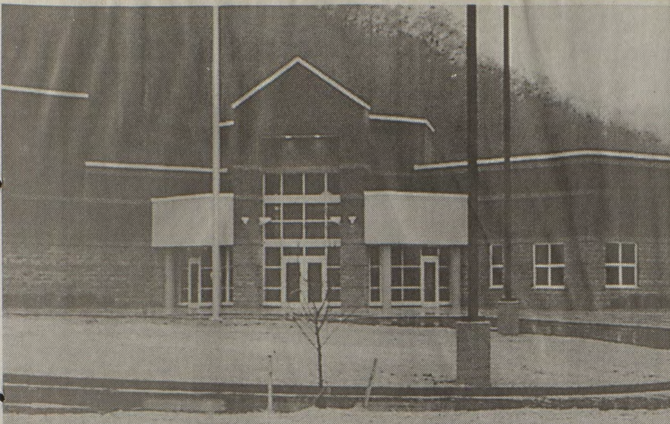
The Martin/Maytown Elementary School is scheduled to open in January after the Christmas break. BellSouth employees worked on the phone lines in the school, and other workers installed the sprinkler system this week. No decision has been made on the name of the school, although a committee has met several times in an effort to select a name for the facility. (photo by Chris McDavid)
