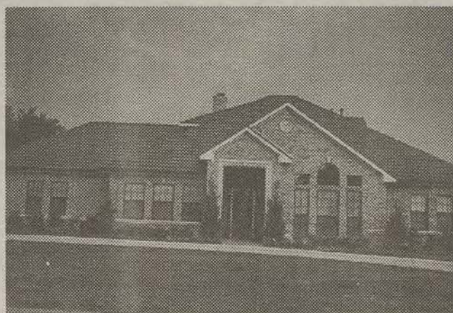
METAL ROOFING PROVIDES many benefits, and it also can be very attractive, like these aluminum shakes.
