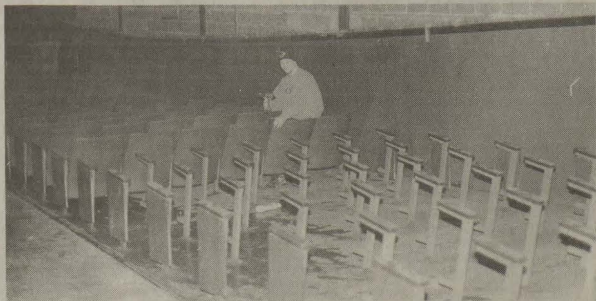
Strand repairs underway
