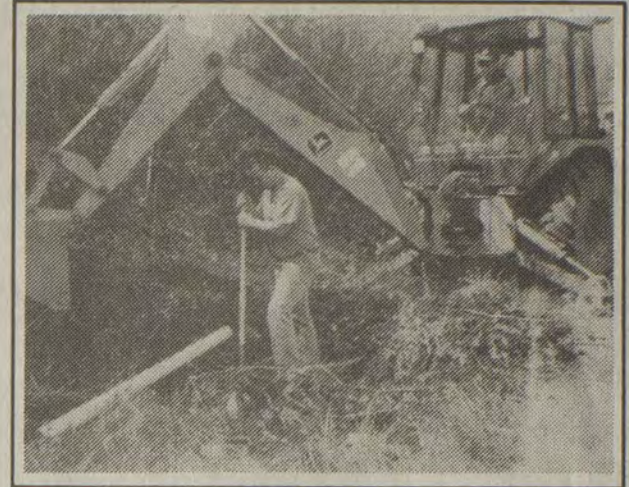
250 MILES OF WATER PIPE
