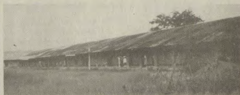
Children of Belize attended this dilapidated wooden schoolhouse.
