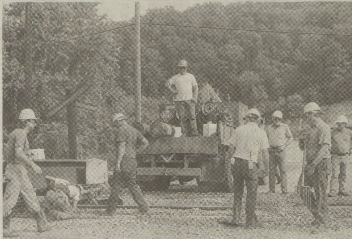
Working on the railroad
