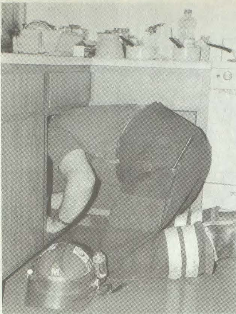
Stop the leak!
