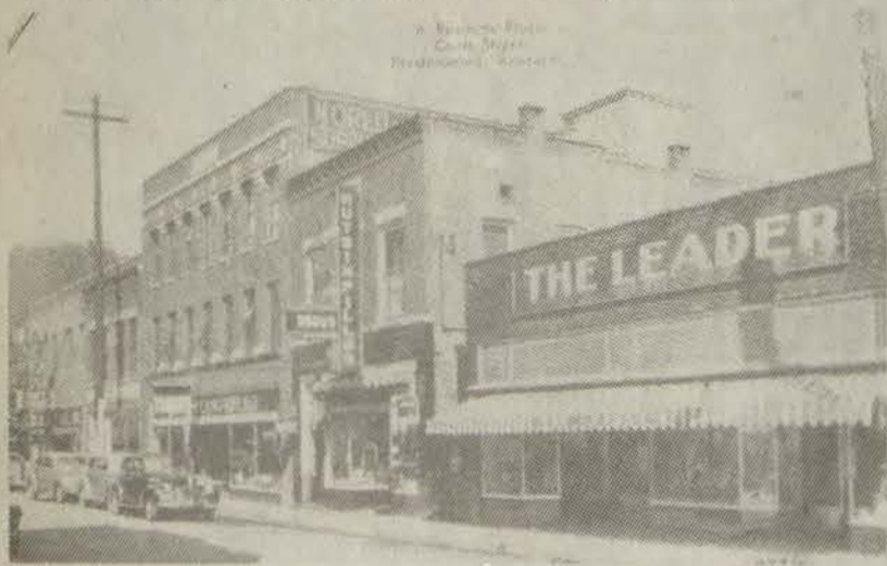
Court Street Prestonsburg
