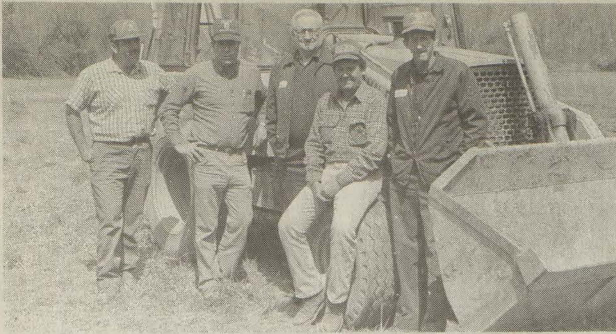
Crew and Equipment Work on Old Drift Park
