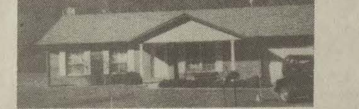
BANNER MAPLE WOOD VILLAGE ESTATES Attractive 3 bedroom, 2 bath home. Central Vacuum system - assumable 8.8% loan. Don't delay in seeing this home.
