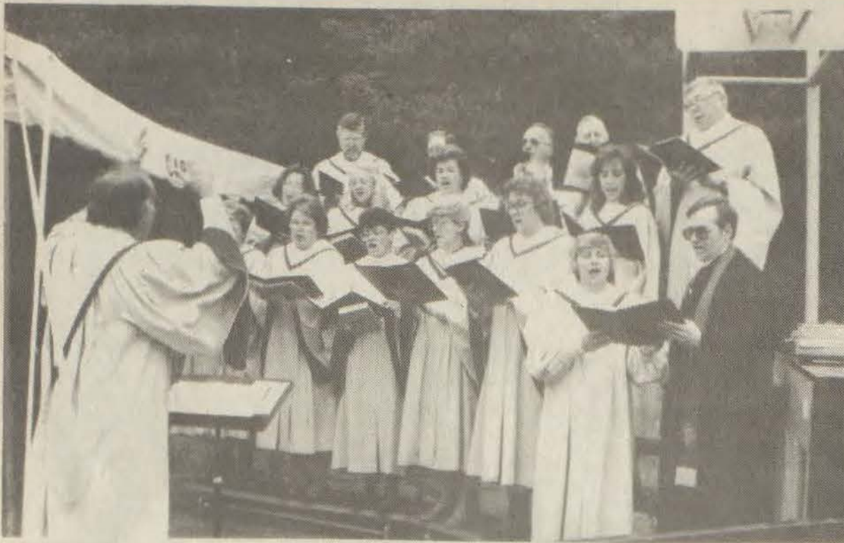
Choir Sings At Ground Breaking
