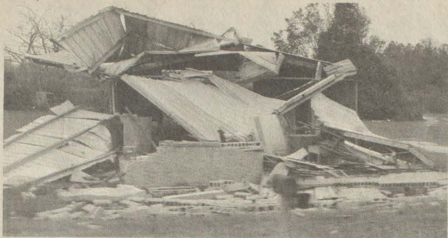
Hurricane Destroys Home
