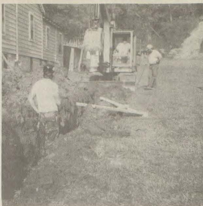
Reclamation Work Begins
