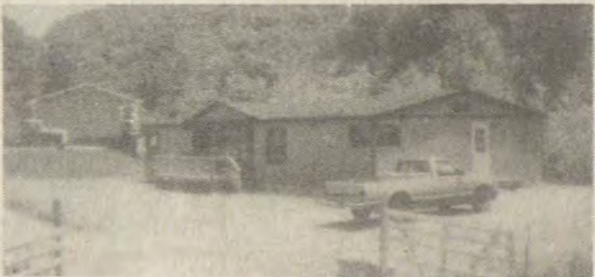
BETWEEN PRESTONSBURG AND PIKEVILLE —Located at Ivy Creek. A new 1500 sq. ft. house that has 3 bedrooms, 2 baths, great room with fireplace, patio and electric heat and air. Situated on a large 125-ft. lot and priced to sell at $55,000. Call today for showing, 874-9033, and ask for Morris.
