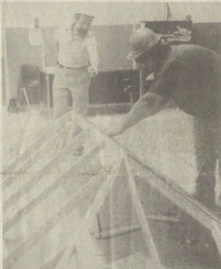
JOB CORPS STUDENT John Miller (right) nails a shingle to a scaled down model of a roof in his afternoon carpentry class while instructor Clay Goebeler lends assistance. The class teaches all aspects of house construction.
