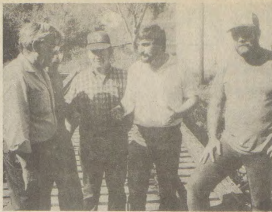
WHEN THE WATER RUNS HIGH, this trestle on which Edsel Moore, Arnold Fitch, Bill Duff, Magistrate Jackie Edford Owens, and Mack Stewart stand, acts as a dam causing Right Beaver Creek to flood low lying areas, nearby.
