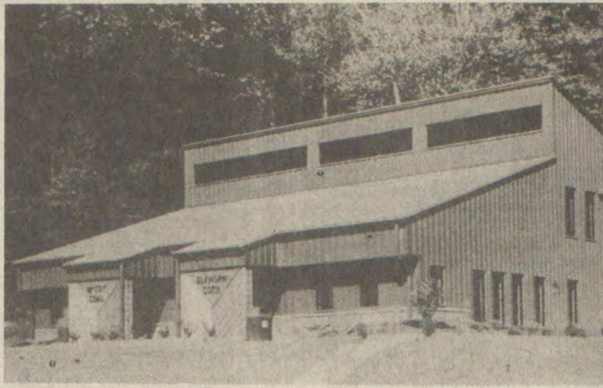
An administrative/engineering building built for McCoy-Elkhorn Coal Corporation in Kimber, has been named to Varco-Pruden Buildings' in 1986 Hall of Fame for excellence in design and construction.
