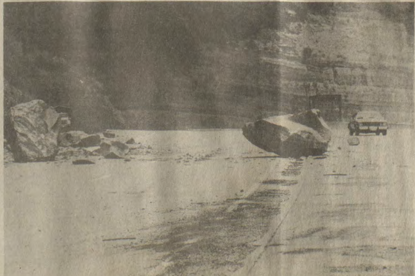
THESE BOULDERS COVERING MORE THAN HALF THE HIGHWAY, presented added hazards to motorists traveling new Ky. 80 at Martin, Saturday. The rockfall blocked two lanes of traffic until its removal several hours later.
