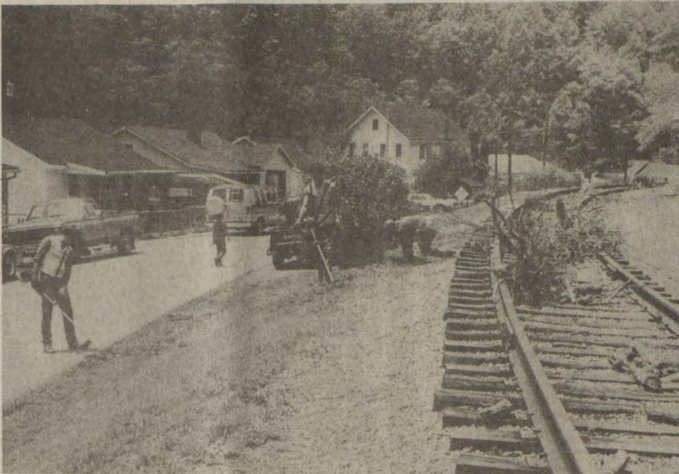
CENTRAL TO a four-week clean-up of Lower Burton has been a youthful crew of workers, including Charlie Martin, left, Gary Day, and Phil Jones, seen here tidying up Friday along the old railroad track. An idle fund once intended for road repairs has been tapped to finance the restoration project.
