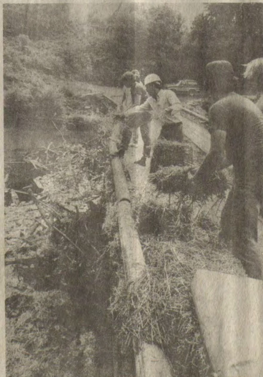
BALES OF HAY were used in an effort to contain an oil spill on Mare Creek last week. A Disaster and Emergency Services crew, assisted by two workers from the state Division of Water, tried for 13 hours to clean up the oil, about 4000 gallons of which polluted Mare Creek and the Big Sandy River following a pipe rupture at the Dannemiller Oil Co. plant.
